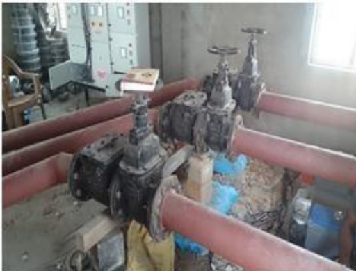
Under Construction pump house
