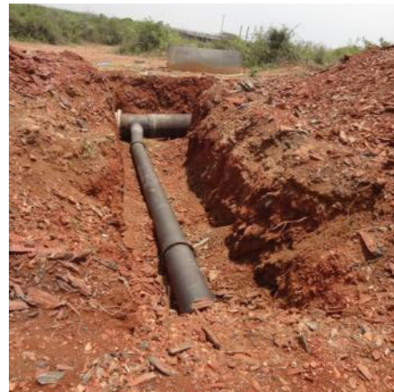
under construction pipe works
