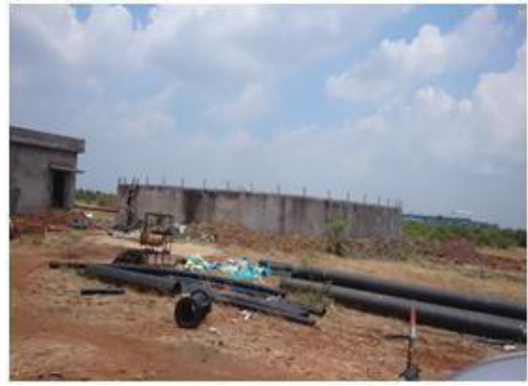
Under construction 2 lakh Gallons GLSR
