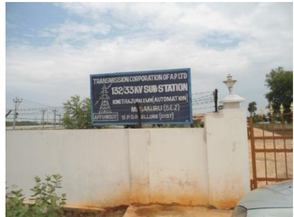
Existing 132/33KV sub-station
