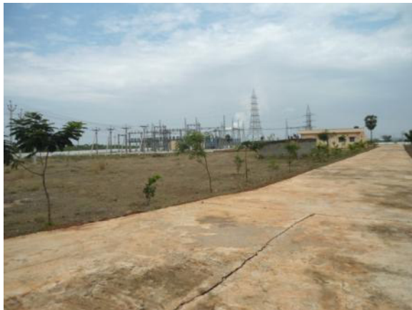
Existing 132/33KV sub-station
