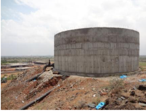
Under construction 4 lakh Gallons GLSR
